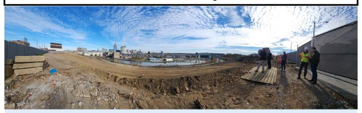
If you've driven down W. 25th or Detroit or sat across the river at Merwin's Wharf, you've likely seen a slight change in Irishtown Bend. Over the course of the initial stabilization phases, more than 60,000 cubic yards of material has been removed off the site (to date). And this Spring, the steel will start to arrive in preparation for the bulkhead replacement along the Cuyahoga River. Stay tuned & take a look from Merwins!
