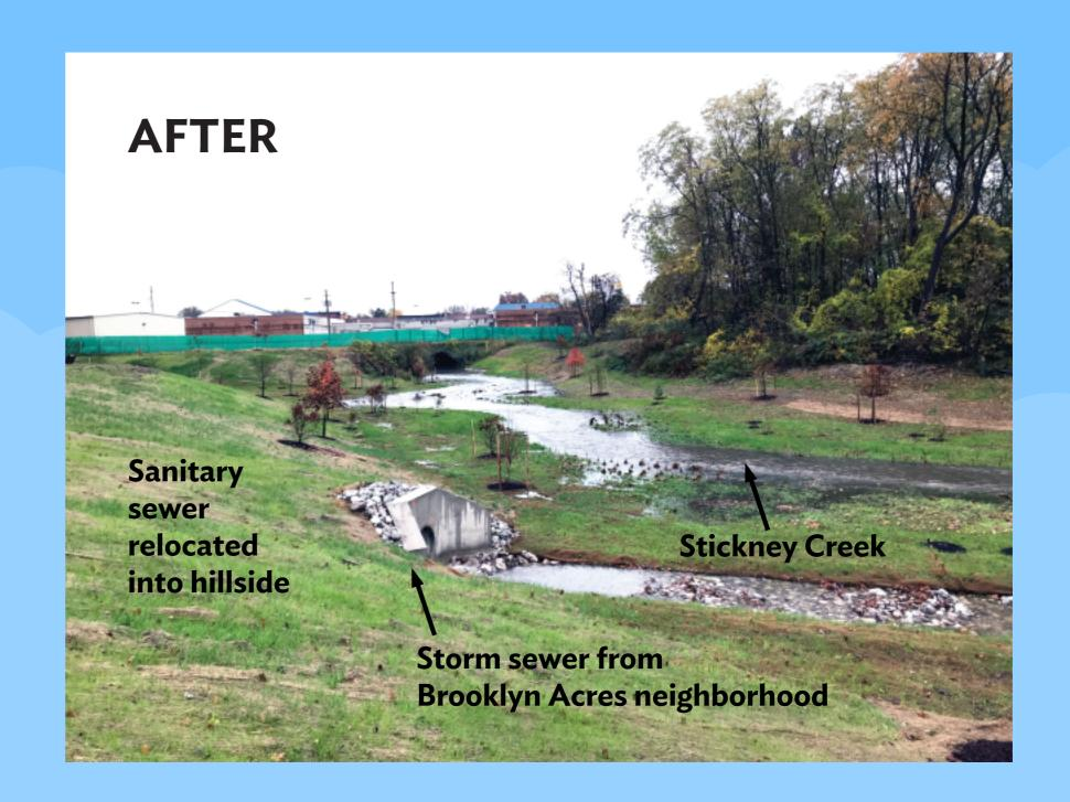
The Sewer District's solution was to move the stream and the sewer away from one another and reconnect Stickney Creek to its floodplain.
